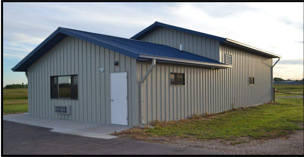
Figure 5: GA Terminal/SRE Building
