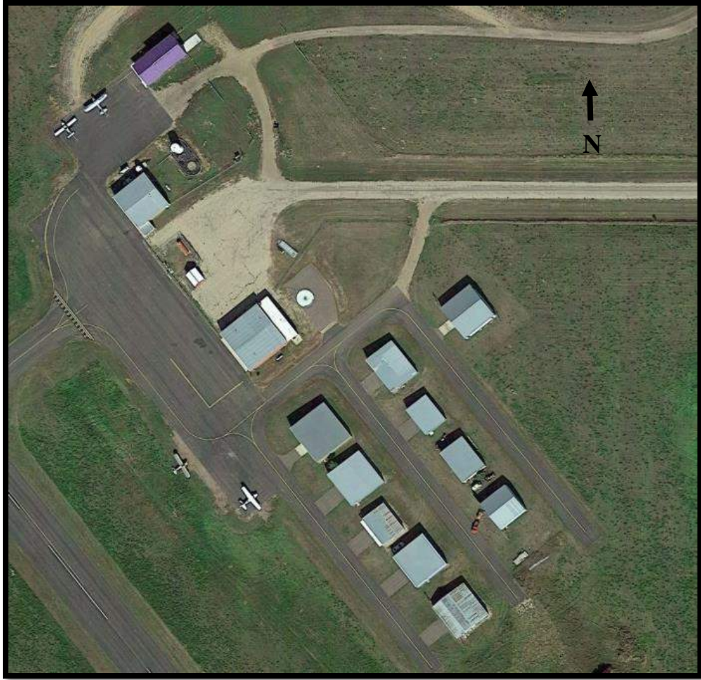
Figure 6: Existing Hangar Area
