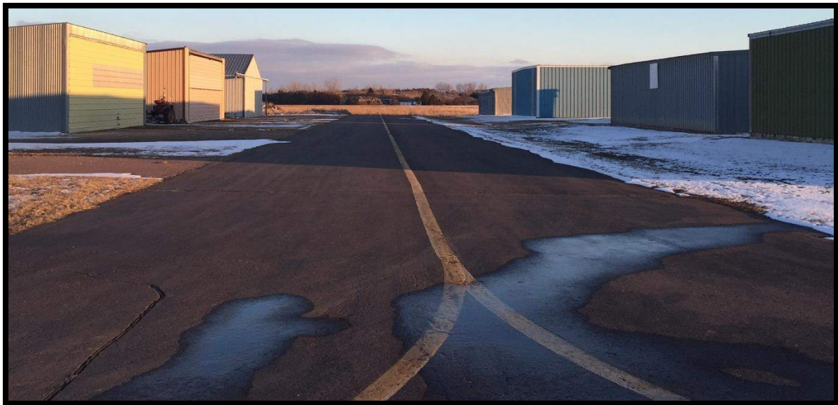
Figure 3: Photo of Hangar Taxilane
